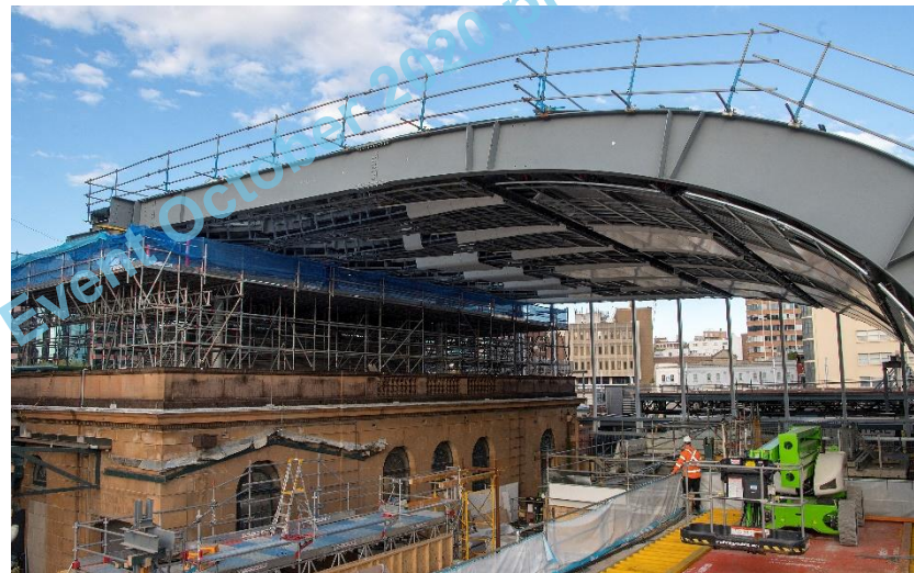
'Hockey sticks' are lifted into place on the new roof over the Northern Concourse at Central Station
