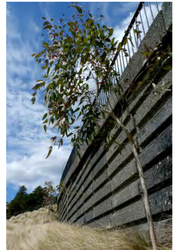
Figure 5.11 Example of a retaining wall in Leura, Blue Mountains, using oxide and an exposed aggregate finish to create a darker effect.
