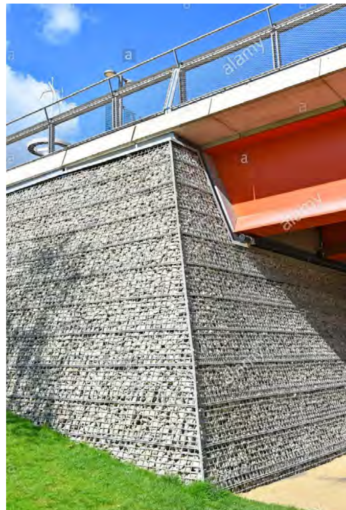
Figure 5.9 Example of a bridge abutment using gabion baskets, giving the structure a more naturalistic character.
