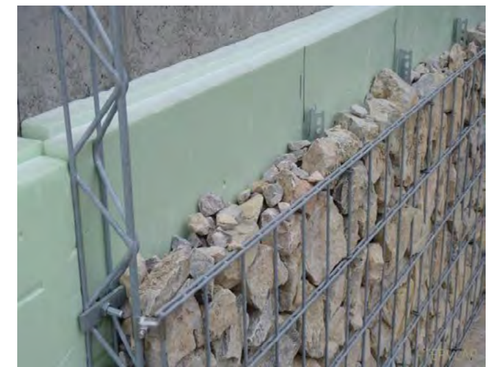
Figure 5.14 Example of a gabion cladding configuration. A similar approach is proposed for the abutment walls.
