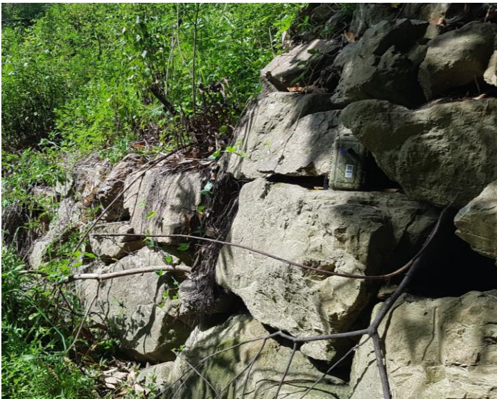
Plate 6 Dry argillite retaining wall adjacent to culvert. Photo facing north west.
