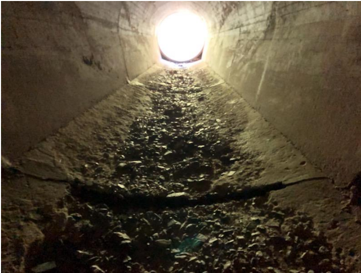
Plate 5 Interior of the concrete pipe, worn from water. Photo facing south east.
