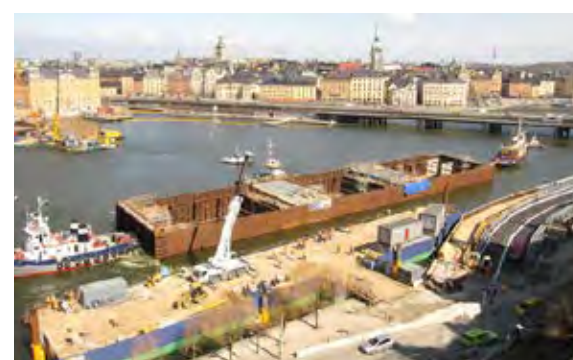
3. Floating steel shell unit arriving at casting facility for concrete construction.
