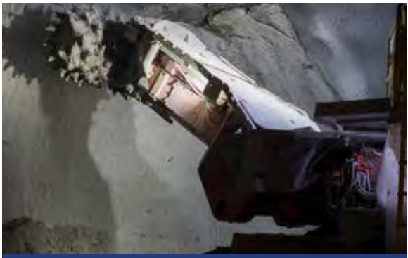
Roadheader tunnelling for M4 East
