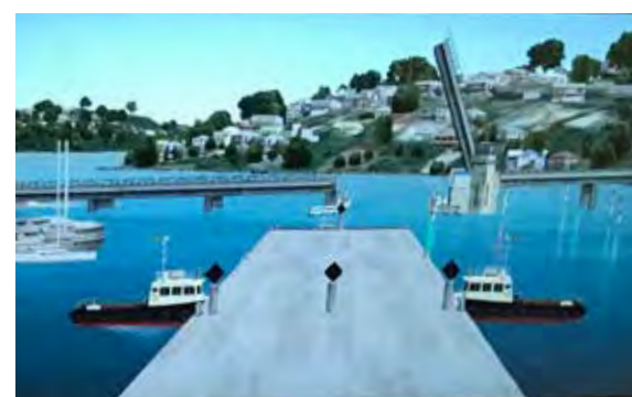
1. Transport of steel shell unit through Spit Bridge.
