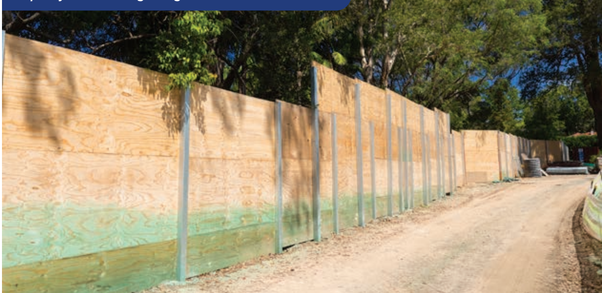
Temporary noise hoarding during construction of NorthConnex
